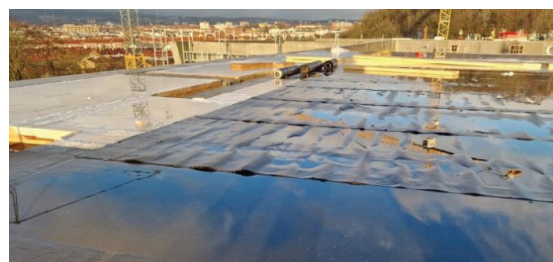
Figure 9: Shows that the bitumen membrane did not bond to the fabric.
