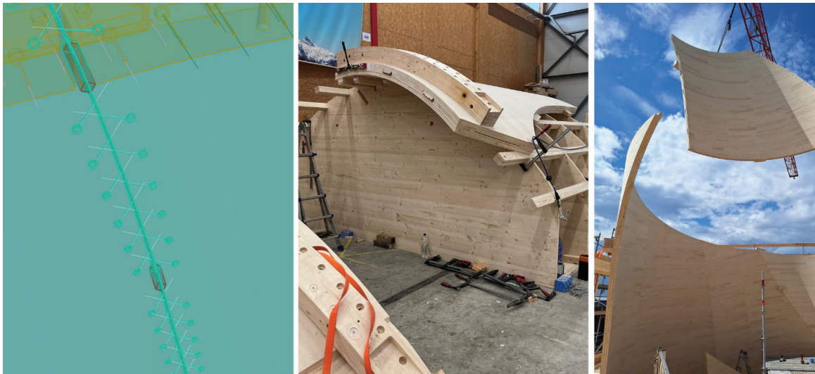
Figure 2. Image of the staircase modelling, pre-assembly of segments in factory hall, and on-site erection. Bertie Hipkin
