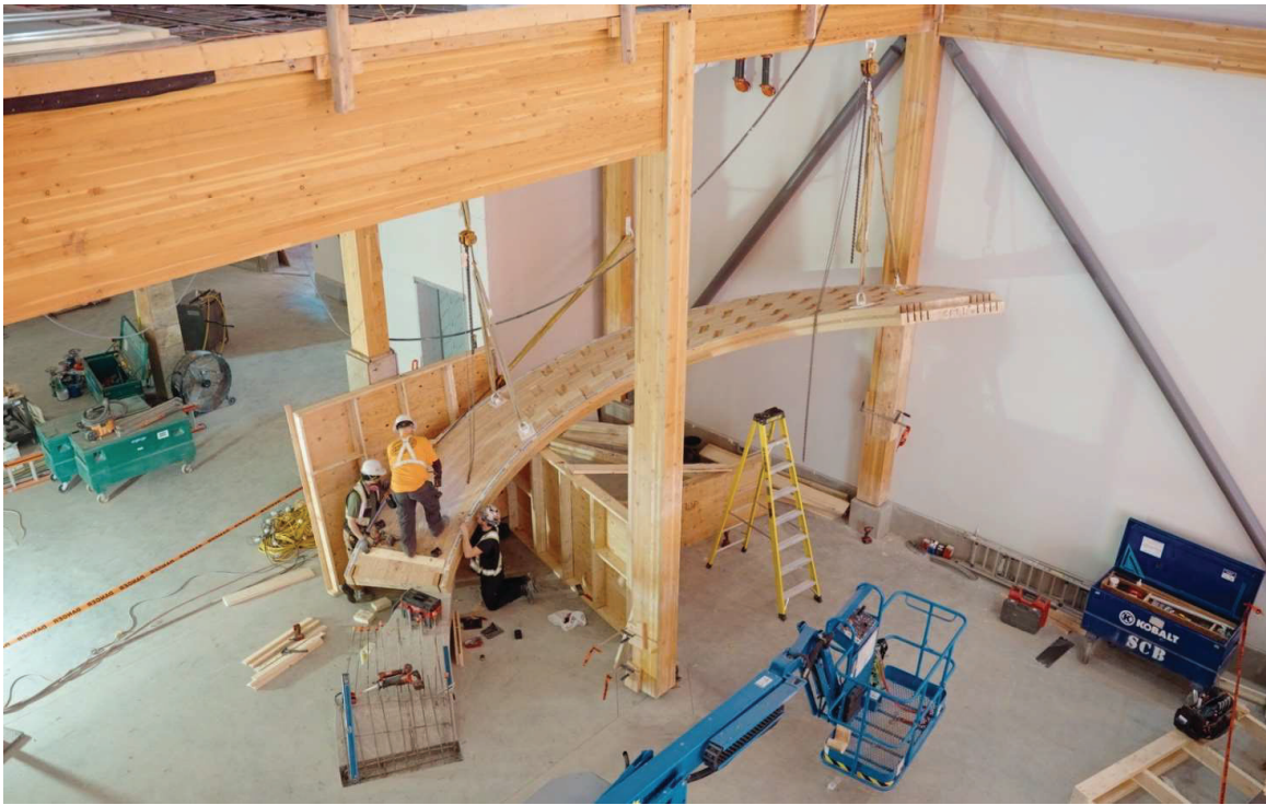
Figure 10: Installation of first CLT half on site using rigging that is attached to existing structure
