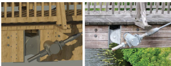
Figure 13. Suspension connection of a timber bridge, as-built model with LoG 400 (left), photo (right) (Images: FHE, Leonard Jordan)
