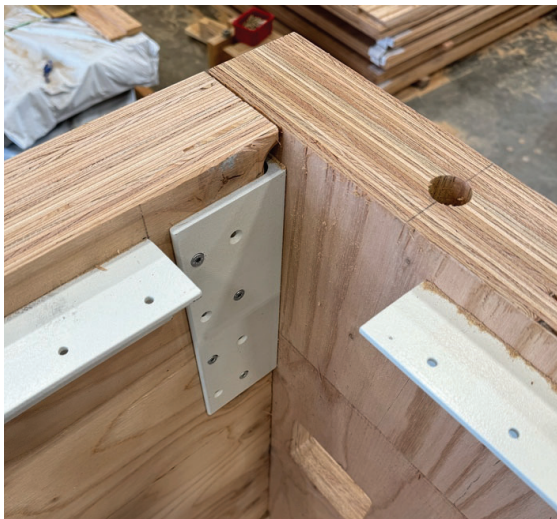
Figure 7. Steel angle connections.
