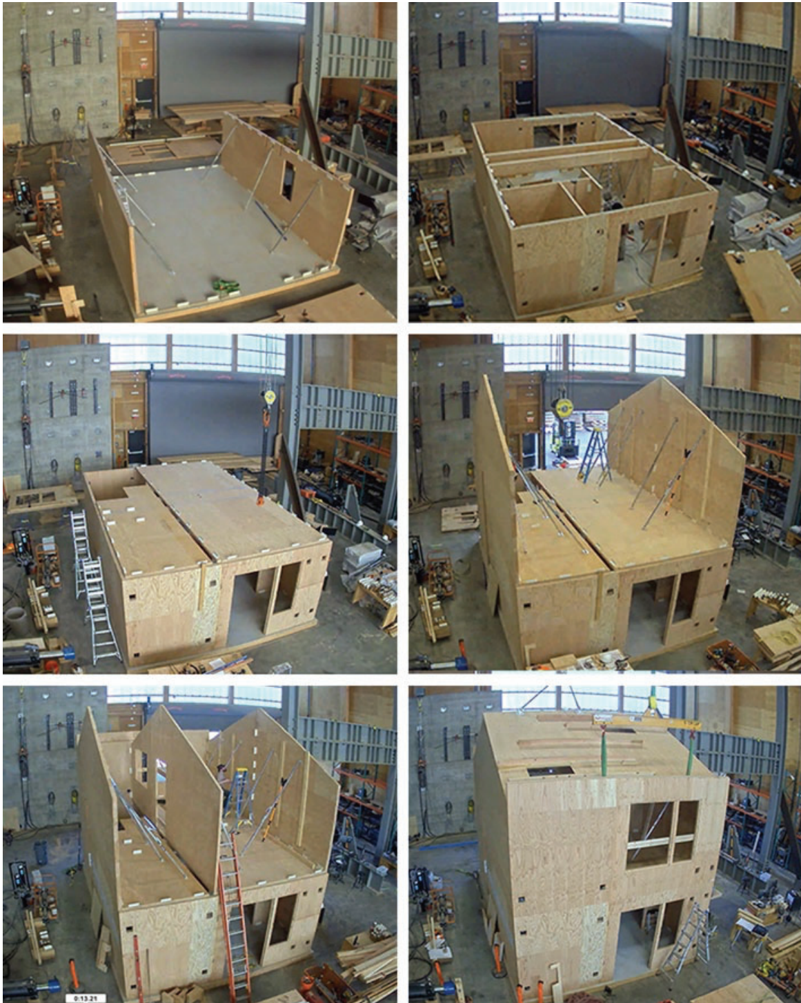
Figure 9. Platform framing assembly sequence. Image: TallWood Design Institute, used with permission.
