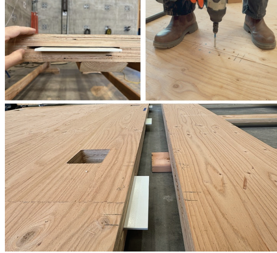
Figure 6. Mortise panel-to-panel connection.
