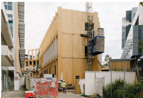
Figure 4: CLT Shear Wall
