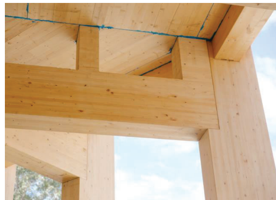
Figure 7: Beam Column Junction with Penetrations for Services
