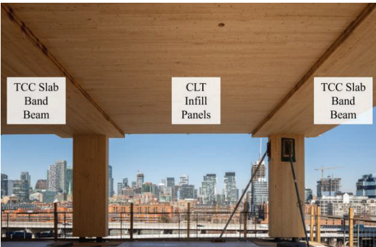
Figure 5. Field test photo of the tested floor system [13]
