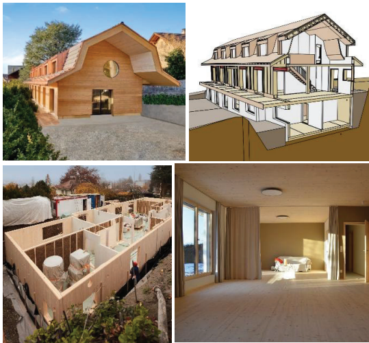
Figure 9. Appartement building in Thun: outside view, visualisation of column and panel construction with TS3, timber basement under construction and interior view of the finished basement (clockwise). Source: www.timbase.com
