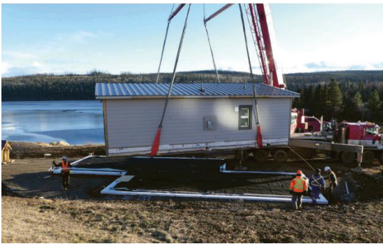
Figure 11. Modular house constructed on a timber slab-on-grade foundation in Canada. Source: www.timbase.com
