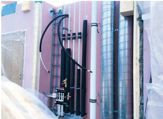
Figure 9. The connection and maintenance of vertical service shaft installations in modular elements are carried out from the stairwell side
