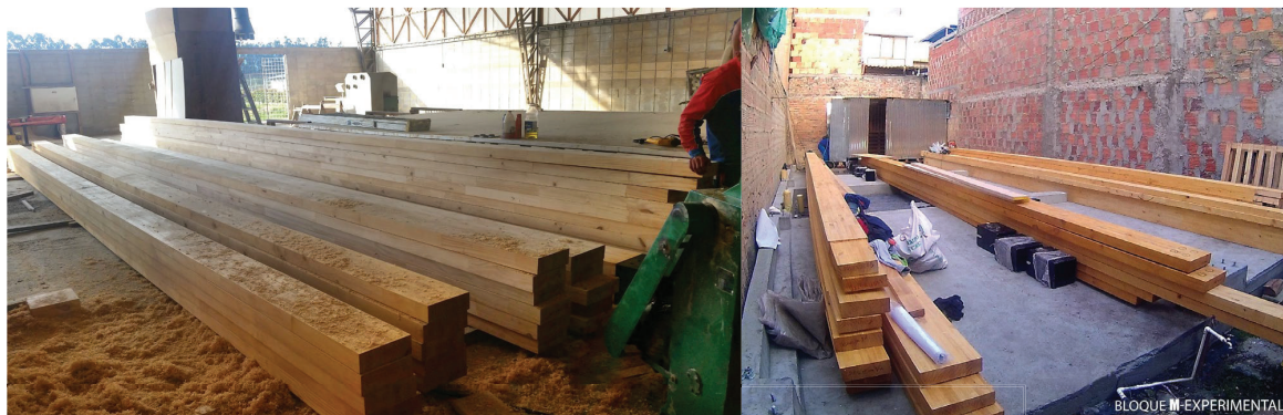
Figure 2. Structural elements in GLULAM at the prefabrication plant and on-site.
