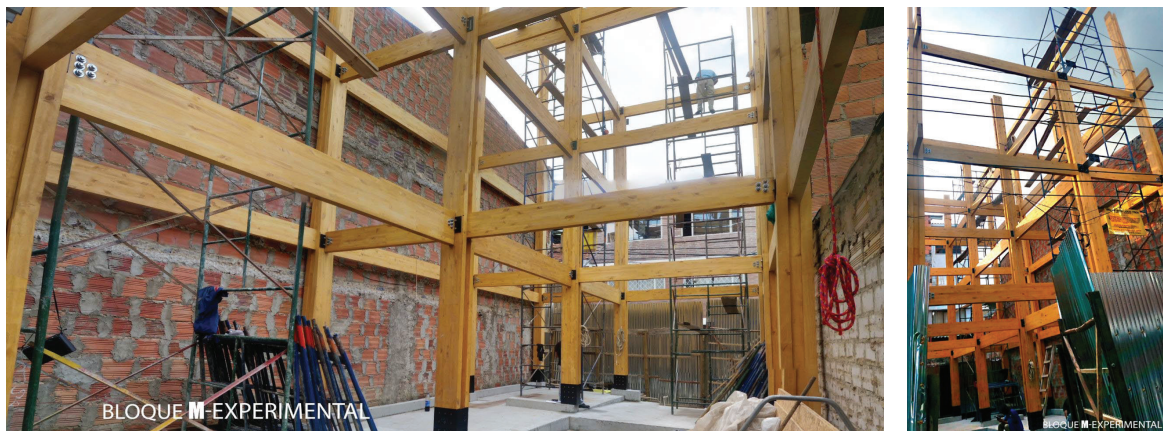
Figure 3. GLULAM Main structure.
