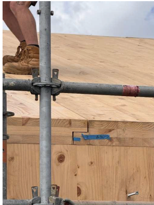
Figure 10. Simple CLT junctions
