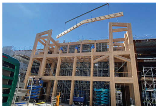
Construction of roof beams
