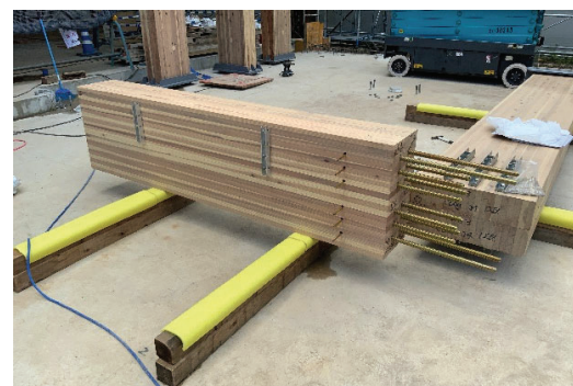
Installation of glued-in-rod (beam)
