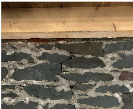
Figure 3. Stone masonry fracturing where hard, cementitious mortar has been used for earlier repairs.
