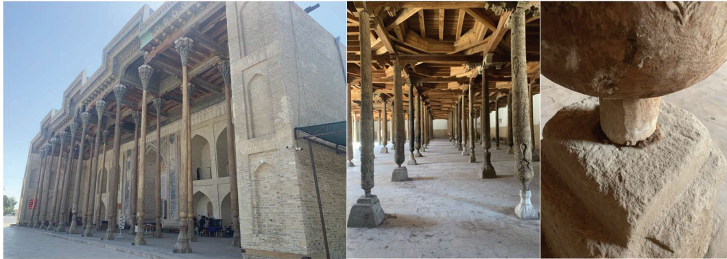
Figure 1. Exterior and interior photos of a 700-year-old mosque in Bukhara, Uzbekistan. The building has URM exterior walls and timber post and beam floor and roof systems. The image at right shows a camel felt pad for seismic isolation at an interior column base.
