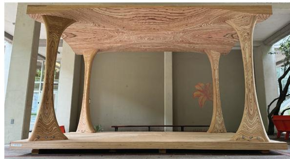
Figure 6. WUP pavilion on 127mm MPP base slab
