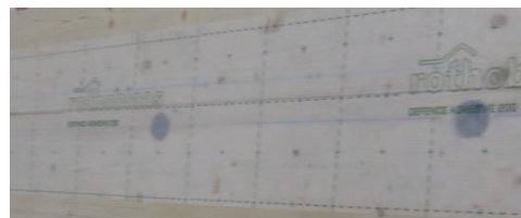
Figure 17. Installation of Defence Adhesive as sealing layer
