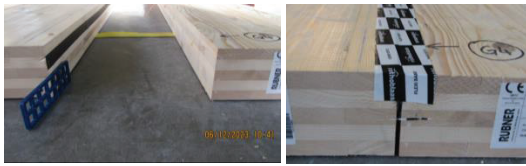
Figure 12. Fire stripe graphite and Flexi Band installed
