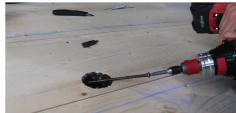
Figure 16. Installation of RING60T
