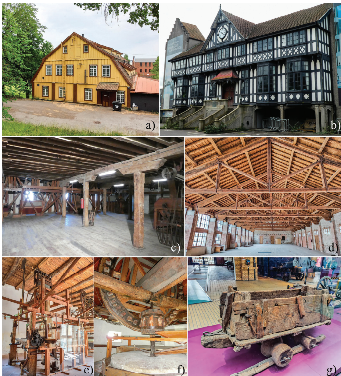
Figure 1. a) Timber structure and cladding facade, Glads Mølle 1736, Norway b) Half-timbered facade, Beamish & Crawford 1919, Ireland c) Post-and-beam, San Antonio flour mill 1852, Spain d) Timber truss, Royal Sawmill of Valsain 1884, Spain e) Silk loom, Italy f) Windmill cogwheels, Spain g) Trolley from Transylvania 1700, Technikmuseum Germany.
