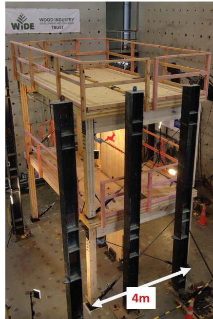
Figure 1b: Full-scale two-story CLT wall structure with resilient rocking walls and resilient tension bracing frame – resilient tension frame direction.
