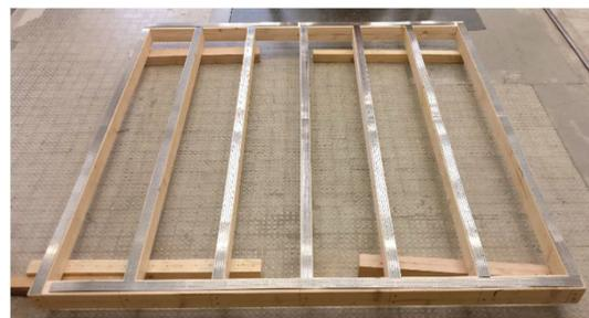
Figure 15: Frame of a wall element with TMF strips applied
