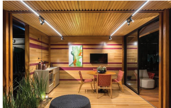
Figure 5: Wood ceiling made of Marupá NLT
