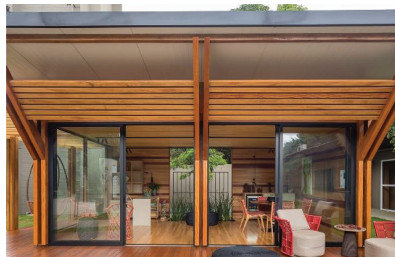
Figure 6: Timber structure is made of Garapeira wood
