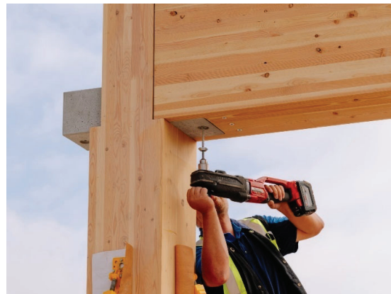
Figure 11 – TCN Installation at Marpole Community Centre
