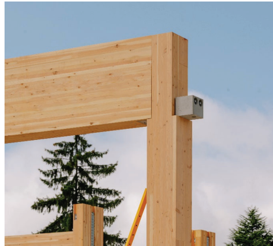
Figure 12 – Installed TCN at Marpole Community Centre
