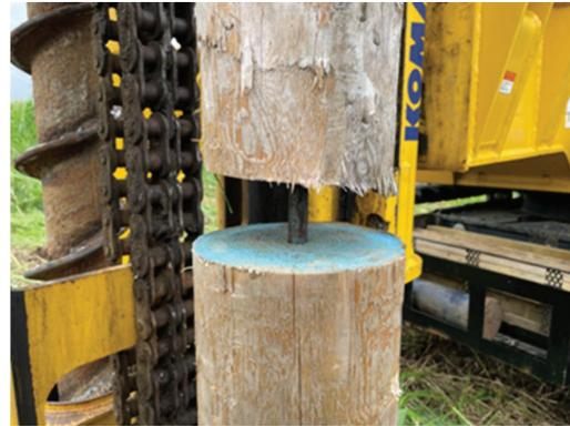
Figure 4 Photograph of joining logs
