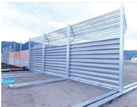
Fig.9: Steel wind-stop type snow fence
