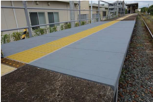
Fig.16: CLT platform at the railway station
