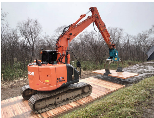
Fig.2: Installation of CLT plates
