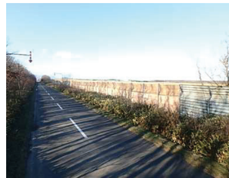
Fig.13: CLT wind-stop type snow fence at the public road
