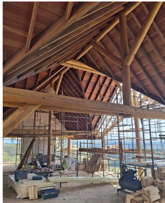
Figure 9: Timber frame and covering details
