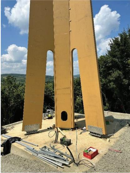
Figure 9. Assembly of the base and wings of the first segment on the reinforced concrete foundation
