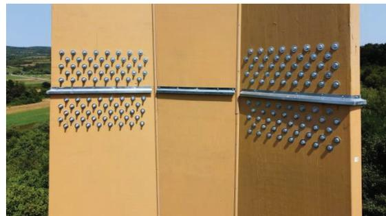
Figure 6. The extension of the pole that transmits the bending moment up to a height of 10 meters.
