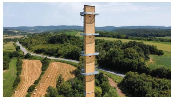
Figure 2. Display of steel assembly platforms for the installation of antenna equipment.
