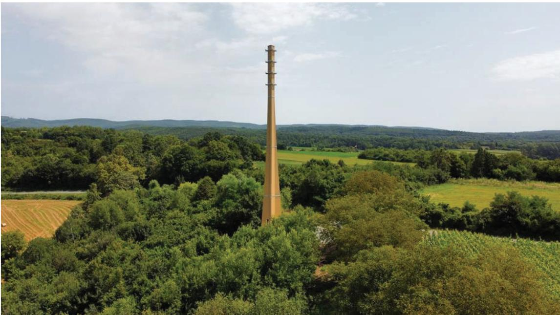
Figure 10. The antenna tower made of glued laminated timber was constructed at the Podcrkavlje location, Croatia.
