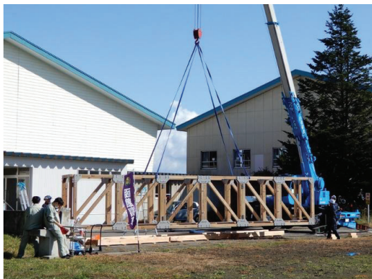
Photo 7. Crane erection
