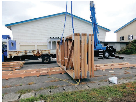
Photo 4. Folded bridge on the erection support
