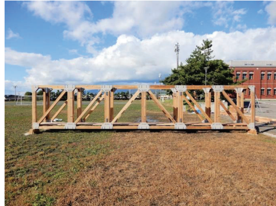
Photo 8. Completion of the bridge erection
