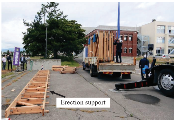
Photo 3. Erection support on the ground
