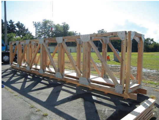
Photo 6. Completion of unfolding work on the erection support
