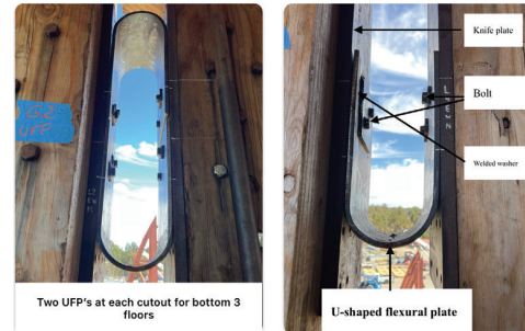
Figure 4: U-shaped Flexural Plate Detail
