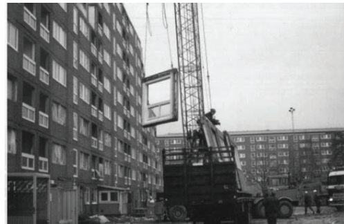
Figure 11: Facade element disassembled at Hammarkullen. (Bengtson, 1997).
