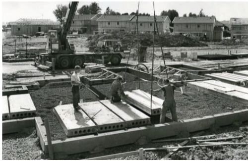
Figure 7: Installation of concrete slabs from Norra Bergsjön at the construction site in Ytterby. (Photo: Lars Mongs, 1985. Used with permission).
