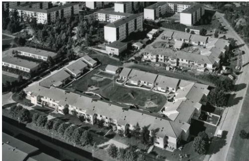
Figure 1: View of the Norra Bergsjön residential area showing the partial deconstruction and conversion into row houses during Phase 2. (Photo: Lars Mongs, 1985. Used with permission).
