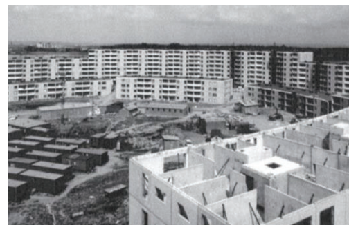
Figure 13: Assembly of precast concrete elements during the construction of the Navestad estate.
