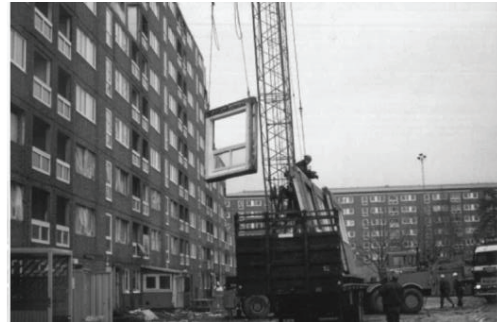
Figure 11: Facade element disassembled at Hammarkullen. (Bengtson, 1997).
