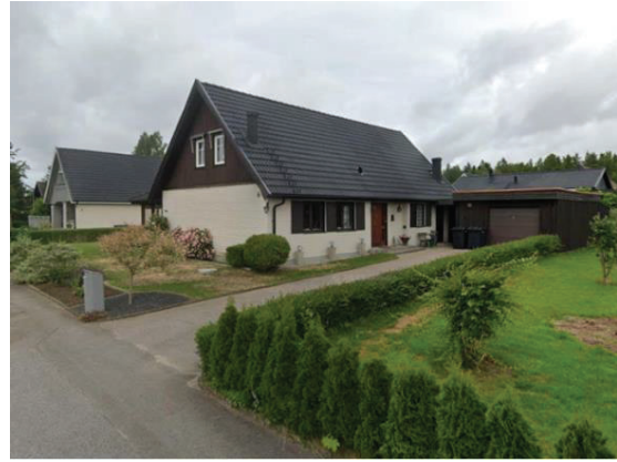
Figure 1: Exterior view of the case study building.
