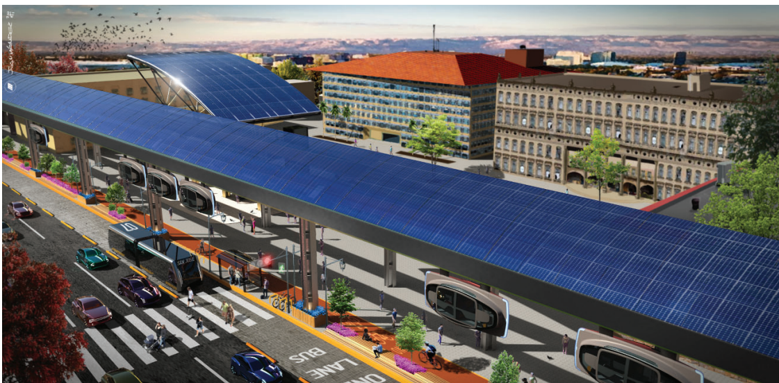
Figure 1: Solar powered automated transit network (ATN) with PV canopy
