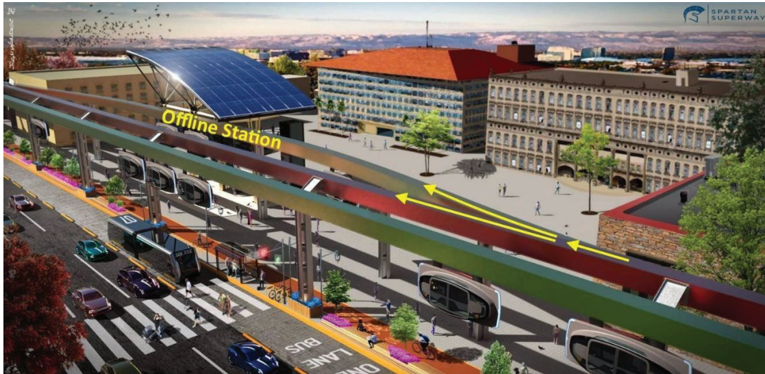
Figure 2: Solar ATN with PV canopy removed to show guideway and offline station
