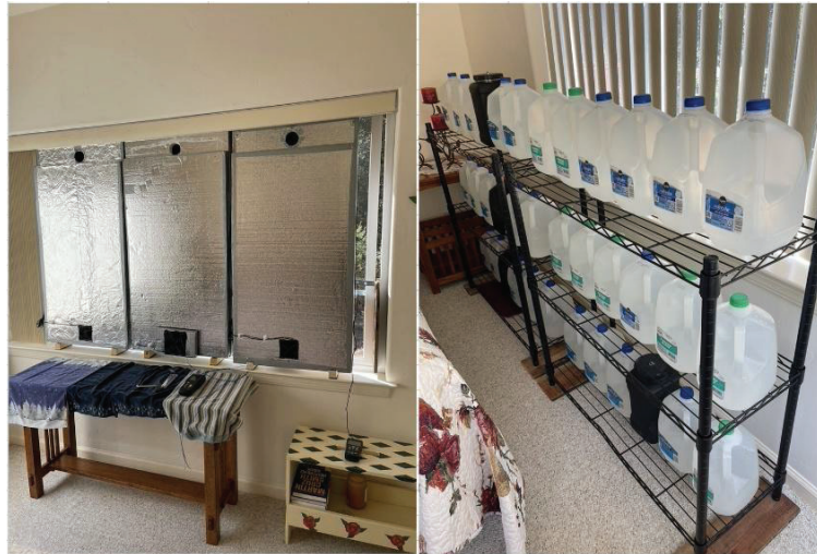
Figure 1. Hot air solar collectors (L) and water thermal storage (R).
